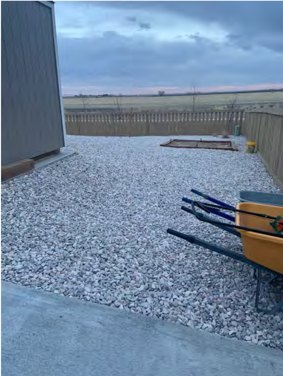
Corner of shed and yard, to demonstrate 6.1% grade
