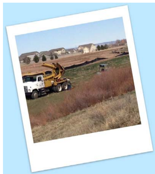
8 Wellington Community Park Phase 1 Construction
