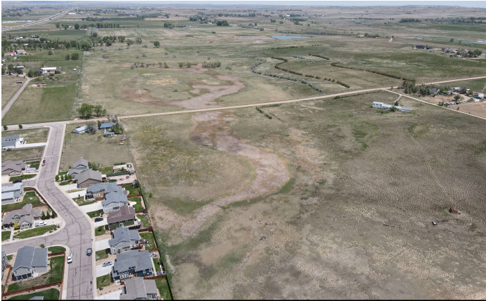
Development has infringed on Wellington SWA Tributary flowpath, which now terminates at the east side of Cotton Park at the Meadows
